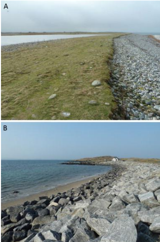
Figure 2. Natural barrier beach in Western Isles, Scotland (A), replaced by rock-armour (B) in an attempt to halt shoreline recession. Examination of A shows gravel on the landward side of the barrier, indicating the barrier is migrating by rolling landward, conserving its sediment volume. The barrier in B is no longer able to do so and the beach that fronts it will eventually suffer coastal squeeze.
