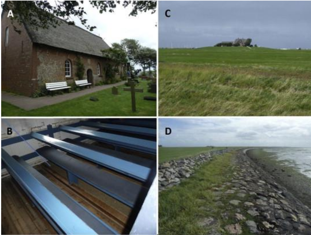
Figure 3. The Halligen of the German Waddensea are remnants of salt marsh on which communities have historically lived with periodic flooding. Historic adaptation to living in this environment with periodic flooding ranged from simple measures such as constructing the floor of the church (A) from wooden boards on top of sand (B) so that flood water could drain easily. More elaborate measures were involved in construction of farms (werfen) on mounds on the marsh surface (C). This enabled the marsh to persist through periodic inundation and sedimentation. This natural resilience is being undermined by construction of dykes (D) to reduce flood frequency. The lower dyke eliminates most summer floods while the upper dyke reduces the frequency of winter flooding. Both have the effect of reducing the sediment input to the marsh surface.
