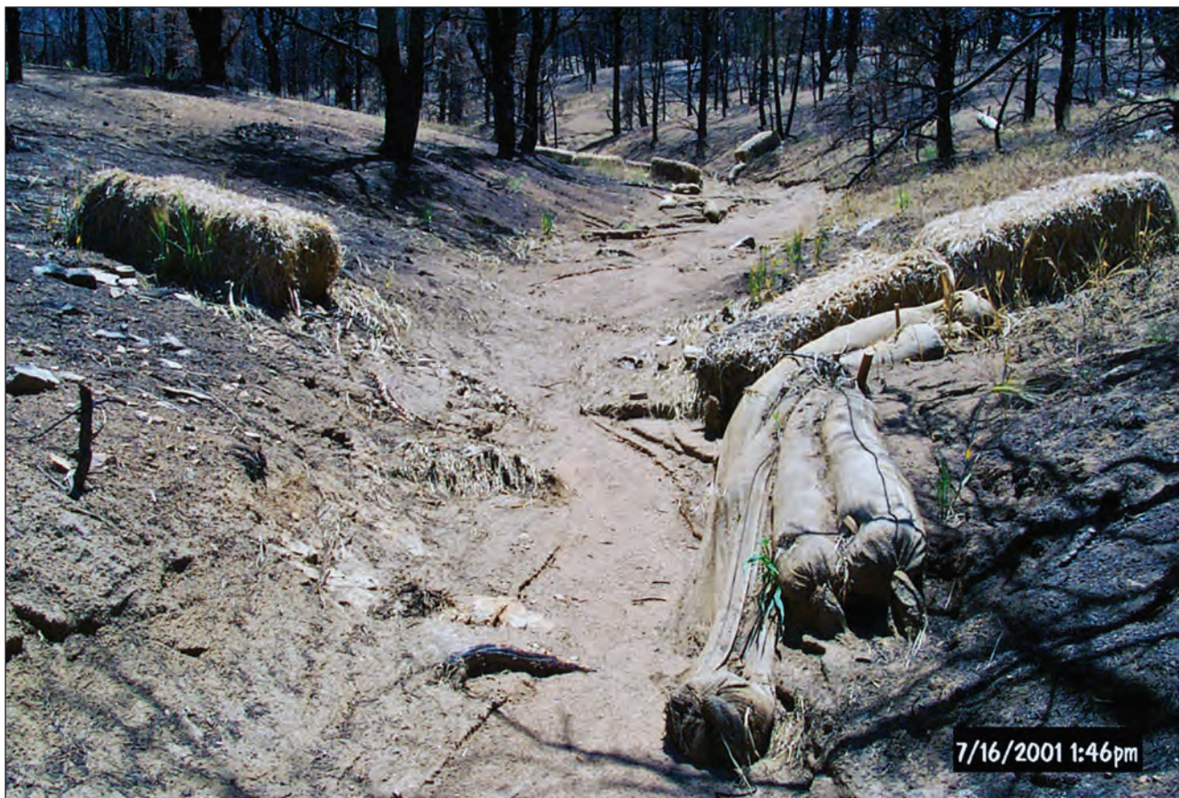
Figure 2—Failure of check dams with straw bales and wattles following an extreme rain event.
